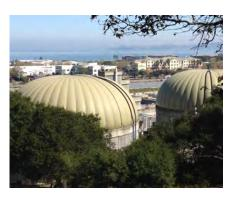
The organic waste is co-digested with wastewater solids in anaerobic digesters to produce additional biogas that is used as fuel in the Agency's cogeneration system. The mixture of food waste, FOG,
